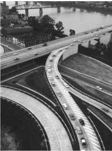
The interstate highways came to serve as informal barriers between communities.
