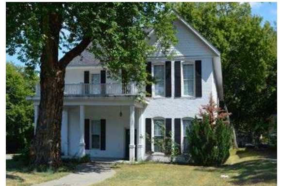
This lovely old home is a sharp contrast to some structures in tract 46 that have fallen into disrepair. Many of the houses in this area are on the National Register of Historic Places.
