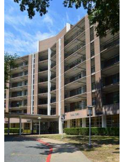
Campus Towers in North Little Rock's tract 28 provides housing for low-income elderly and disabled residents.
